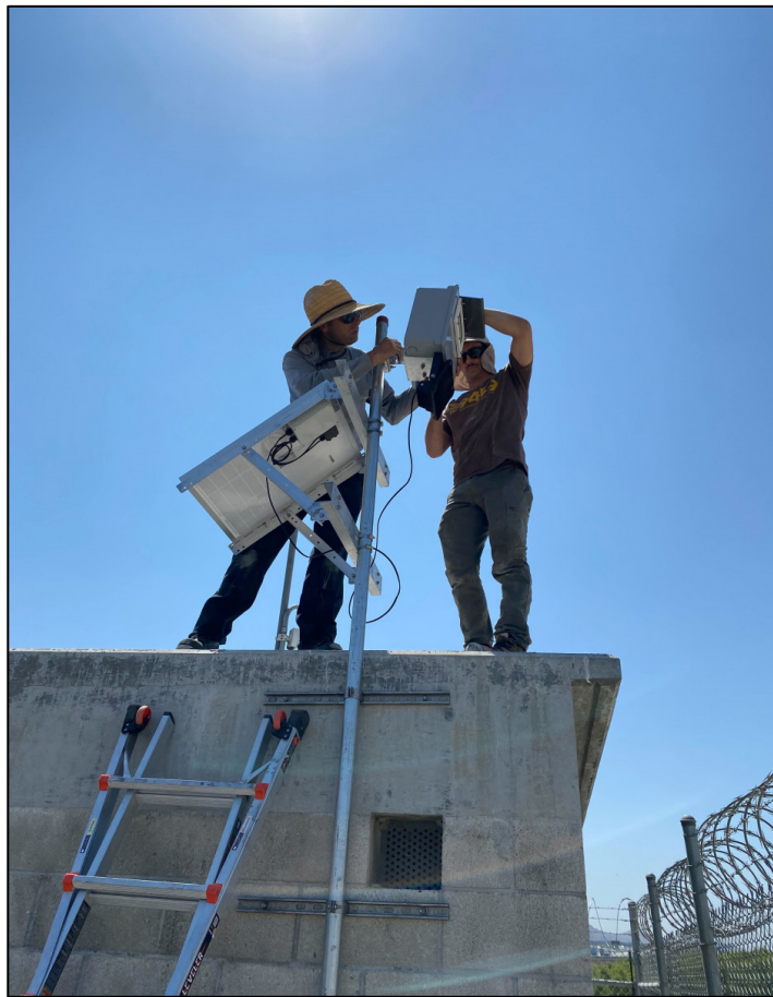
Figure C-29. CVSG, security enclosure, IR illuminator, and solar panel were attached to the 1.5" mast using U-bolts.
