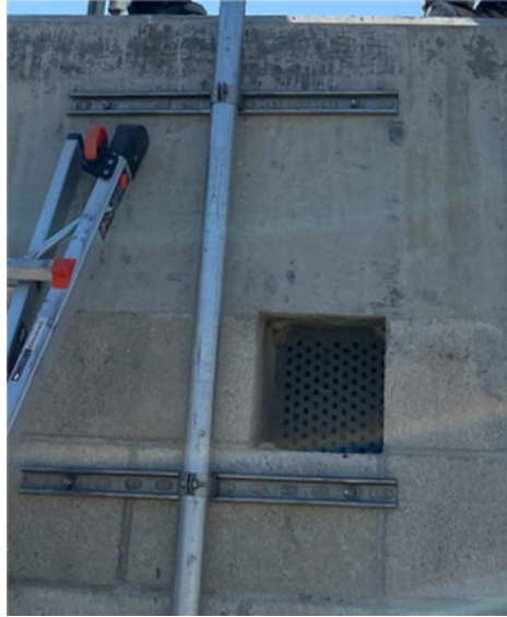
Figure C-28. Strut channel was attached to the USGS gage house using \frac{3}{8} " concrete anchors. Conduit clamps were used to attach the mast to the gage house strut channel.
