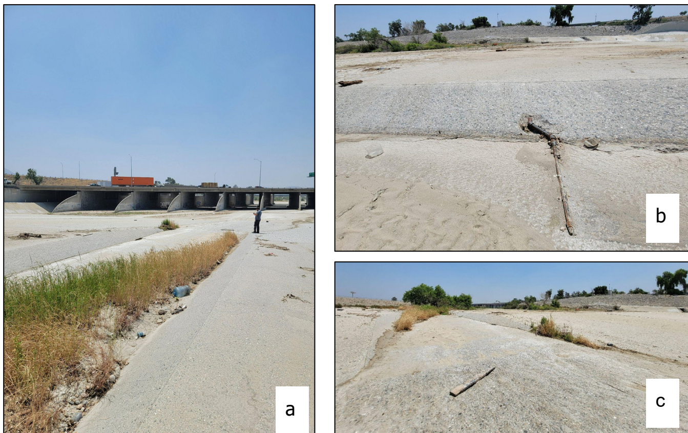
Figure C-54. (a) USGS E Street low-flow channel downstream view. (b) USGS E Street low-flow channel bubbler. (c) USGS E Street low-flow channel looking upstream.
